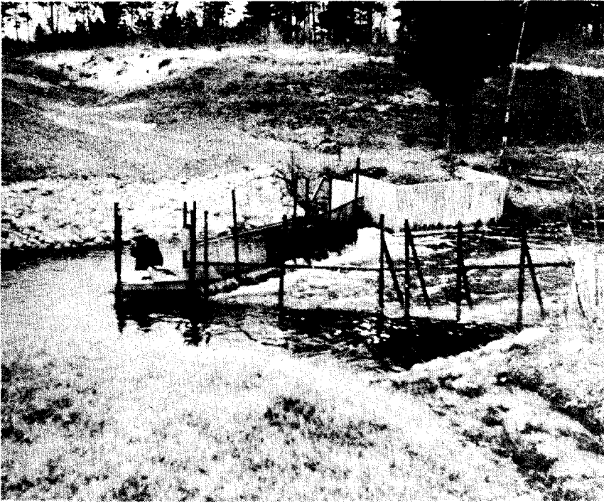
Figure 8.--Carp Creek weir, May 5, 1947. Note damming action of weir screen prior to cleaning. This screen had been cleaned six hours earlier.
