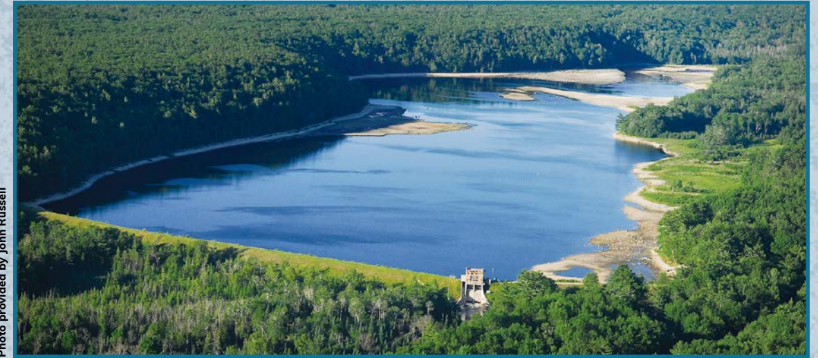
Due to an inadequate spillway, two drawdowns were required exposing the heavy sand filling Brown Bridge Pond prior to dam removal. (Summer 2010)
