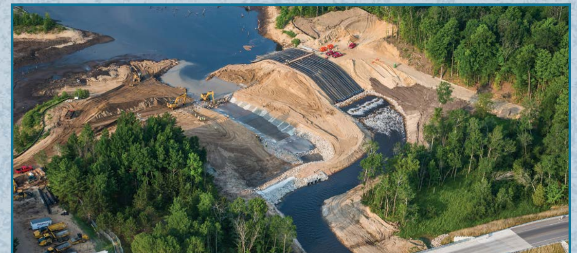
Gravity-fed siphons lowered the impoundment 21’ and an auxiliary spillway (left) drained the remaining water so the siphons could be removed and the river channel built in their place. (July 2017)
