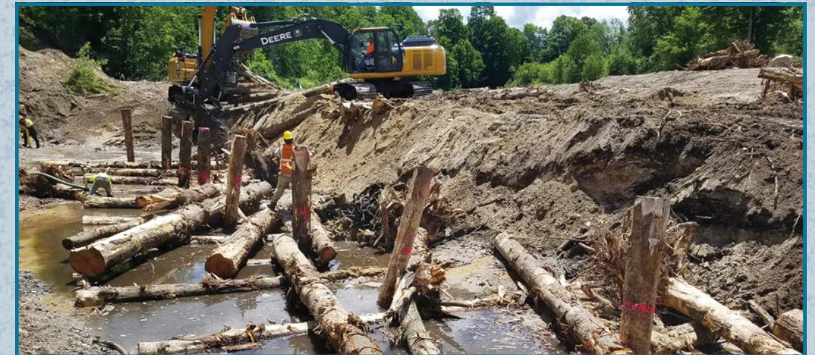
Logs and intact roots are recessed into streambanks and secured to the stream bottom to provide habitat and strengthen outside bends. (June 2017)
